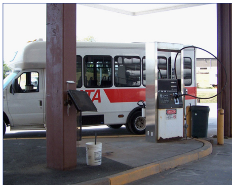
CATA's CNG fueling station.
